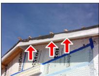
(2) The roof needs compete evaluation/replacement due to damaged battens/blocking, damaged/deteriorated underlayment, loose/damaged fasteners and overall sun damage.
