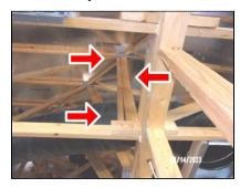
(12) Nailing missing the mark noted at several roof sheathing locations.
