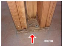
(8) Framing fasteners need securing.
