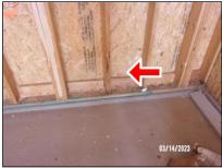
(2) Missing nails at the bearing point straps.
