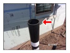
(2) Missing nail guard(s) at the large garage gas pipe.
