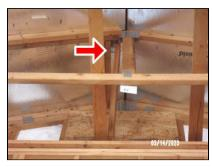
(5) Extra wood should be removed at the east large garage wall.
