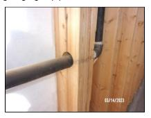
(3) Rust/corrosion noted at the pipes/straps at the water softener and water main.
