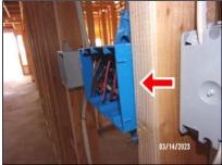
(2) Damaged attic outlet box noted.
