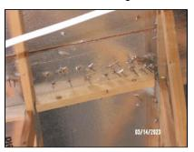
(13) Missing nail guards at the water heater pipes.
