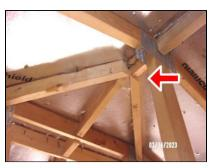
(17) SW large garage stud does not fully connect with the sill plate.
