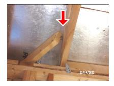
(19) Damaged stud at the east laundry room should be replaced.
