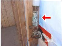
(4) Loose/unsecured water heater flue cover noted.
